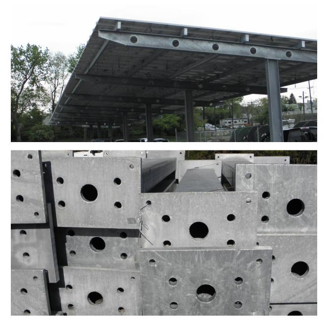
Figure: Hot dipped galvanized steel components with weep holes that allow galvanize to coat inside and out
